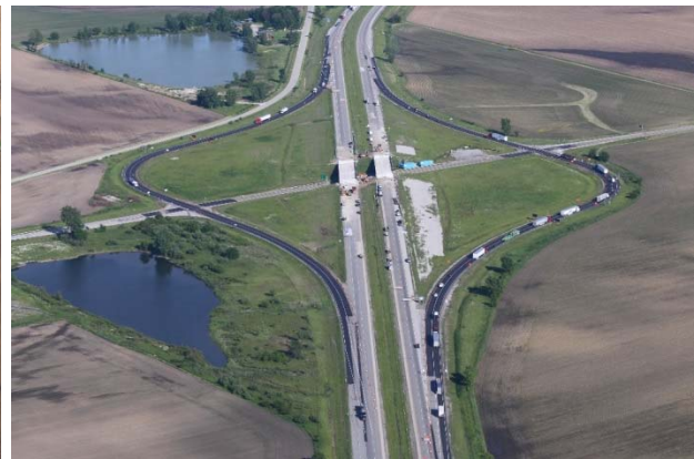
c) Aerial Image During Construction
