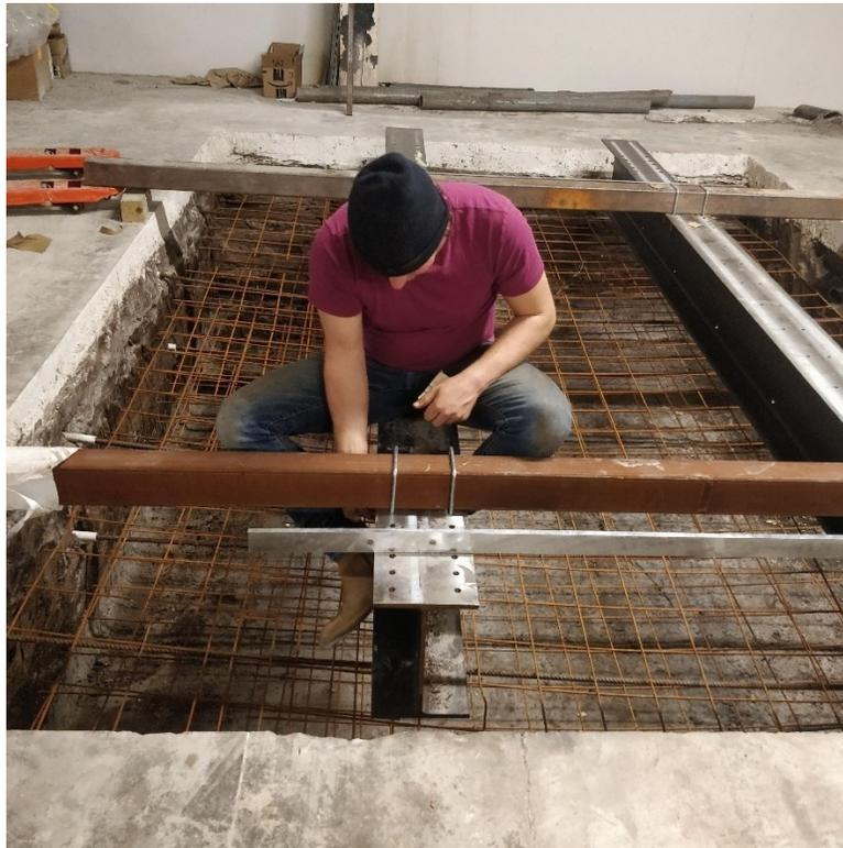
*Figure 23: Preparation of Foundation for Concrete Slab*
